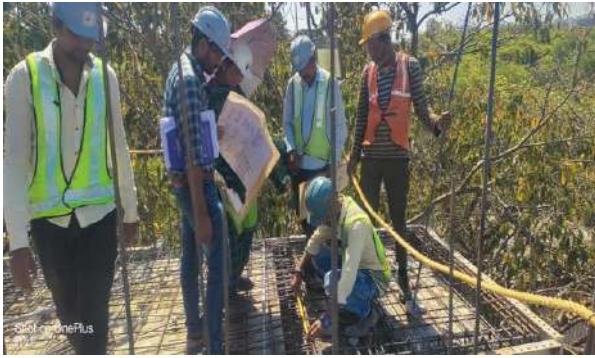
Construction of Additional Infrastructure at IISc Main campus, Bangalore
