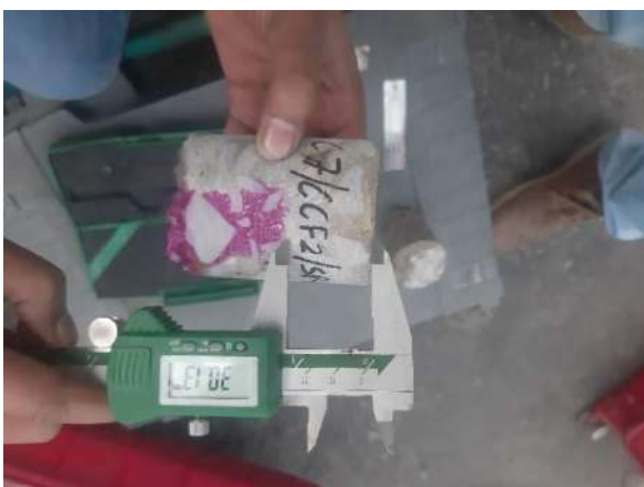
Carbonation depth being measured on freshly extracted concrete core at a Hospital Building site
