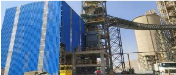
Consultancy services for installation of tyre chips for M/s Oman Cement Company, Oman
