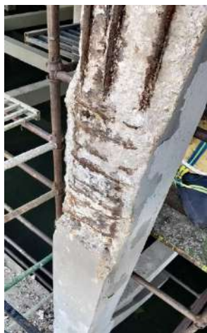
Chipping completed in a selected column at a project site
