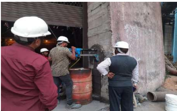
Condition Assessment of RCC Structures at NTPC Tanda
