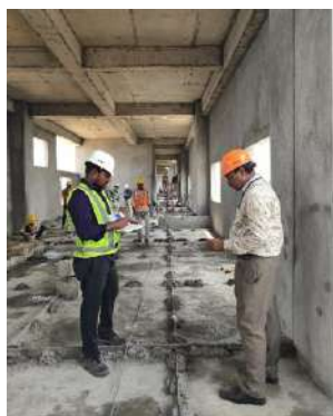
Construction of Additional Exhibition and Convention Hall TNTPO, Tamil Nadu
