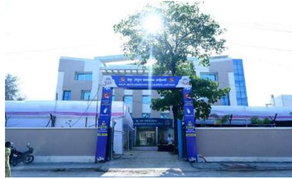
Construction of CBI Building, PUNE
