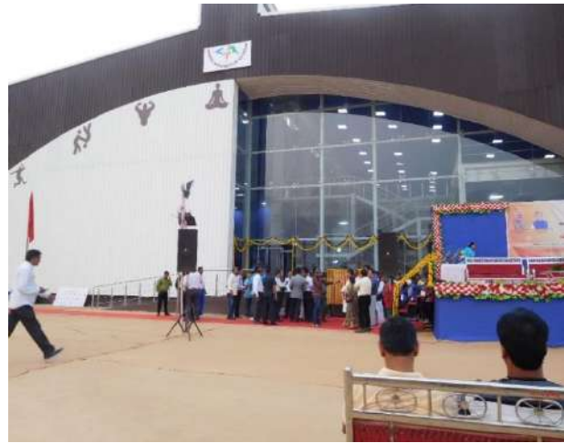
Indoor Multipurpose Hall at Vaghodia (Vadodara)
