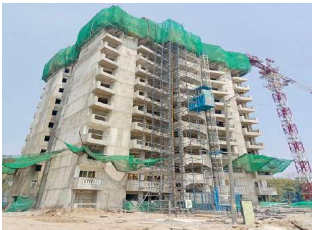
General Pool Residential Accommodation at Kasturba Nagar, Delhi
