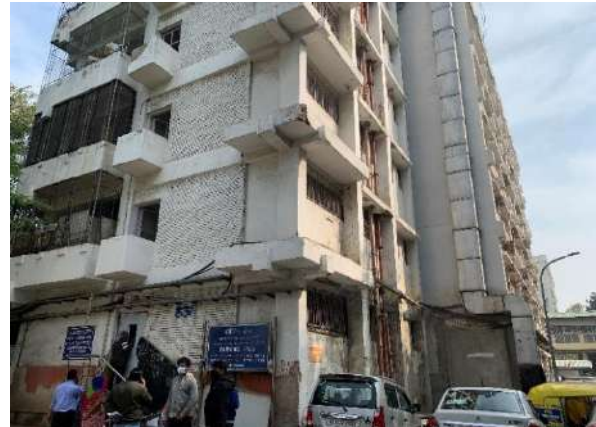
Project site of condition assessment work at RML Hospital New Delhi
